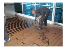
SIS-440 Deck Sealant is a one-part, paste-like neutral cure caulk which, when exposed to moisture in the air, reacts to form a tough, flexible solid rubber compound. The sealant does not sag during cure, and has excellent temperature stability and chemical resistance when cured. Because the sealant is neutral cure, it is non-corrosive to all substrates.
